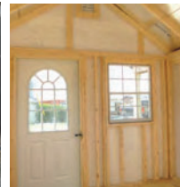
Tyvec Interior Walls
